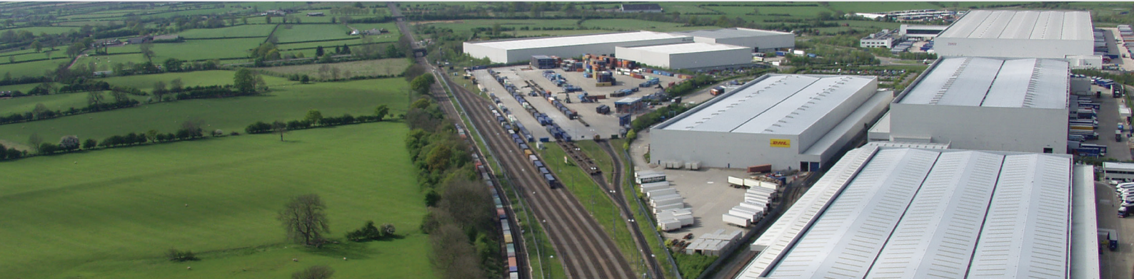
The Davenport International Rail Freight Terminal; a modern SFRI
